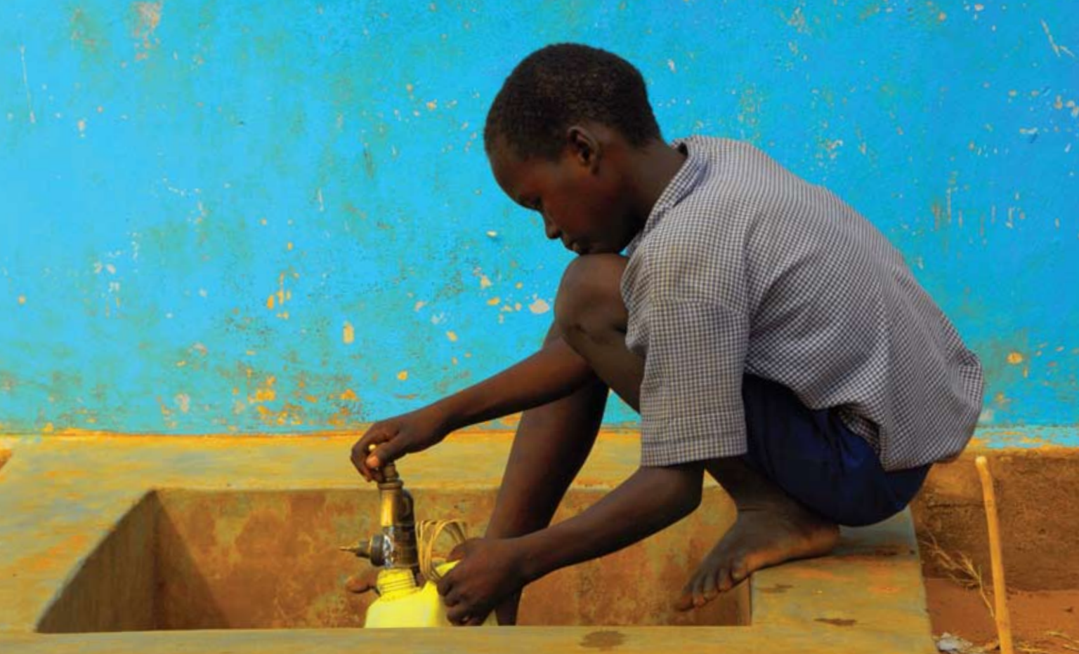
Naturally-occurring springs can be protected with a concrete encasing as a preventative against microbial contamination.
