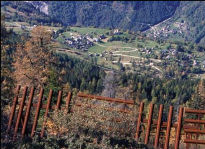
Steel-girded protection constructions in the fraction zone of an avalanche (Braggio, Switzerland). © by Brigitte Wolf.
